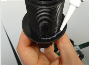
16. Using the silicone provided, make a small bead around the back of the bulkhead flange.
