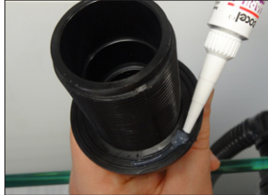
17. Now thread on the rubber washer and again place a bead of silicone around the back of that.
