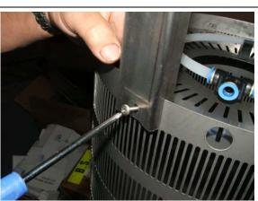
9. Connect the new backwash air tube to the "Eazy" aeration ring
