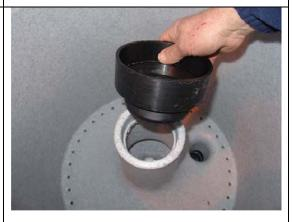
4. Using template supplied cut corner off then fold over line and align with the top of the Nexus inner chamber overflow. Then drill 3x 4mm holes through the Nexus drilling from the inside chamber
