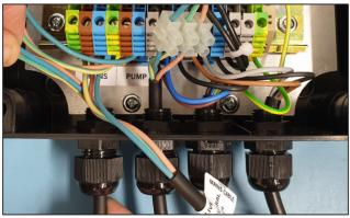
5. MAINS CABLE: Feed enough wire through the gland nut, into the control box to allow you to make the connections to the MAINS terminal block.
