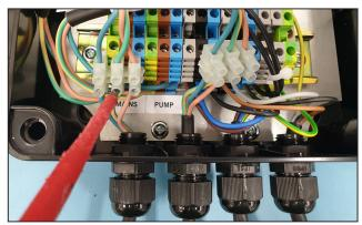
6. Fit the corresponding LIVE, EARTH and NEUTRAL wires into the matching terminal labelled MAINS and tighten with a screwdriver. Now re-fit the lid.
