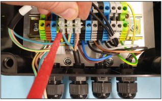
4. Fit the corresponding LIVE, EARTH and NEUTRAL wires into the matching terminal labelled PUMP and tighten with a screwdriver.
