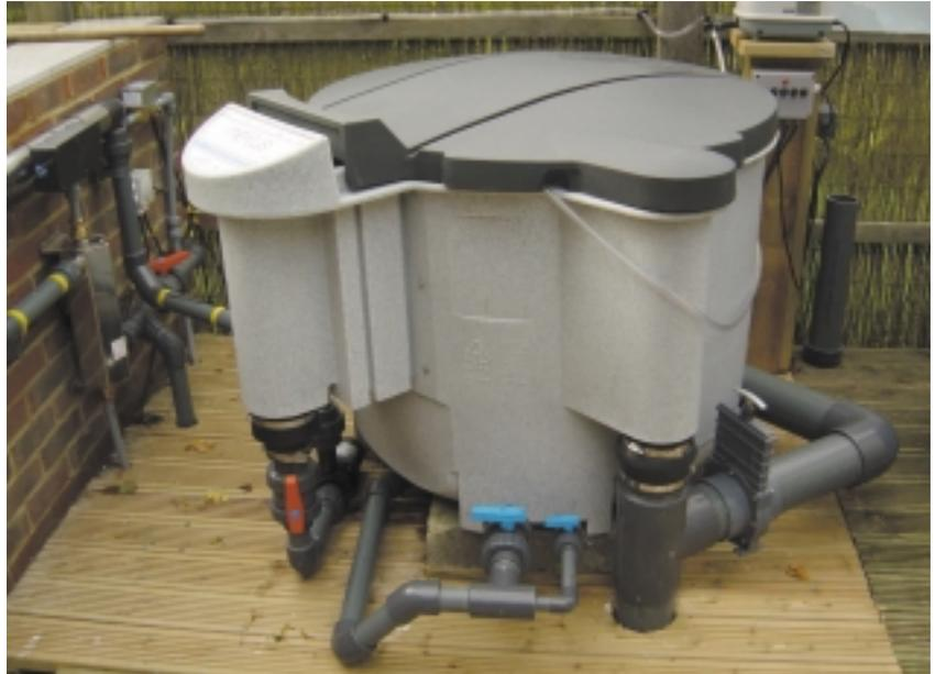
intended, but on the external side of the wall, fit a 90 degree bend and short piece of pipe upwards to the top of the pond wall. The length of this pipe can be adjusted once the filter has been positioned and is running to get the water level absolutely right – once the level is established, the pipe fittings can be glued in place. Overflows can of course also be fitted into a filter, but we did not want to cut any more holes in the Nexus!
